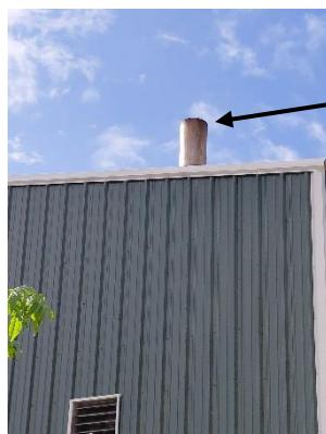
Light colored haze was spewing from the stack during every blowdown sequence in the pollution control system (PCS) which lasted about 2 to 3 mins. The blowdown sequence occurs every 7 mins.
