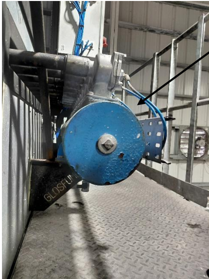
Main Manifold for the blowdown high pressure air supplies
