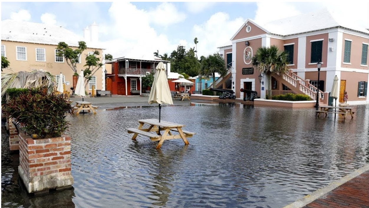
Flooding in Town Square, St. George is predicted to increase with climate change. Photo: Bernews. October 2017
